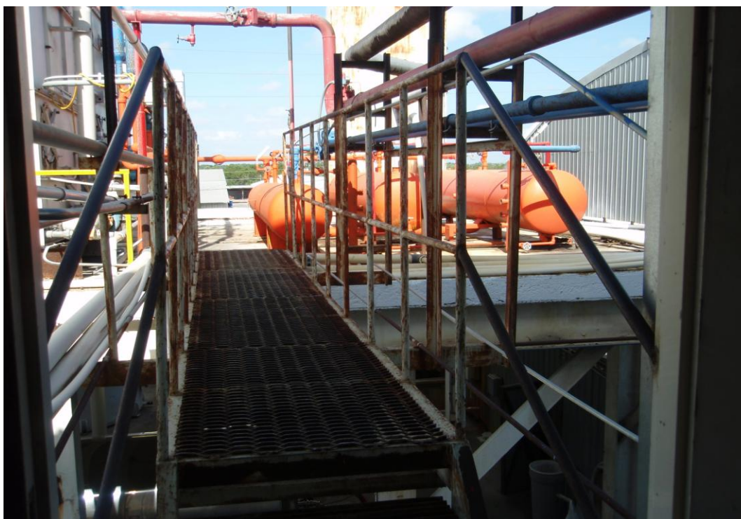
Ammonia storage tanks on site, used for refrigeration.
