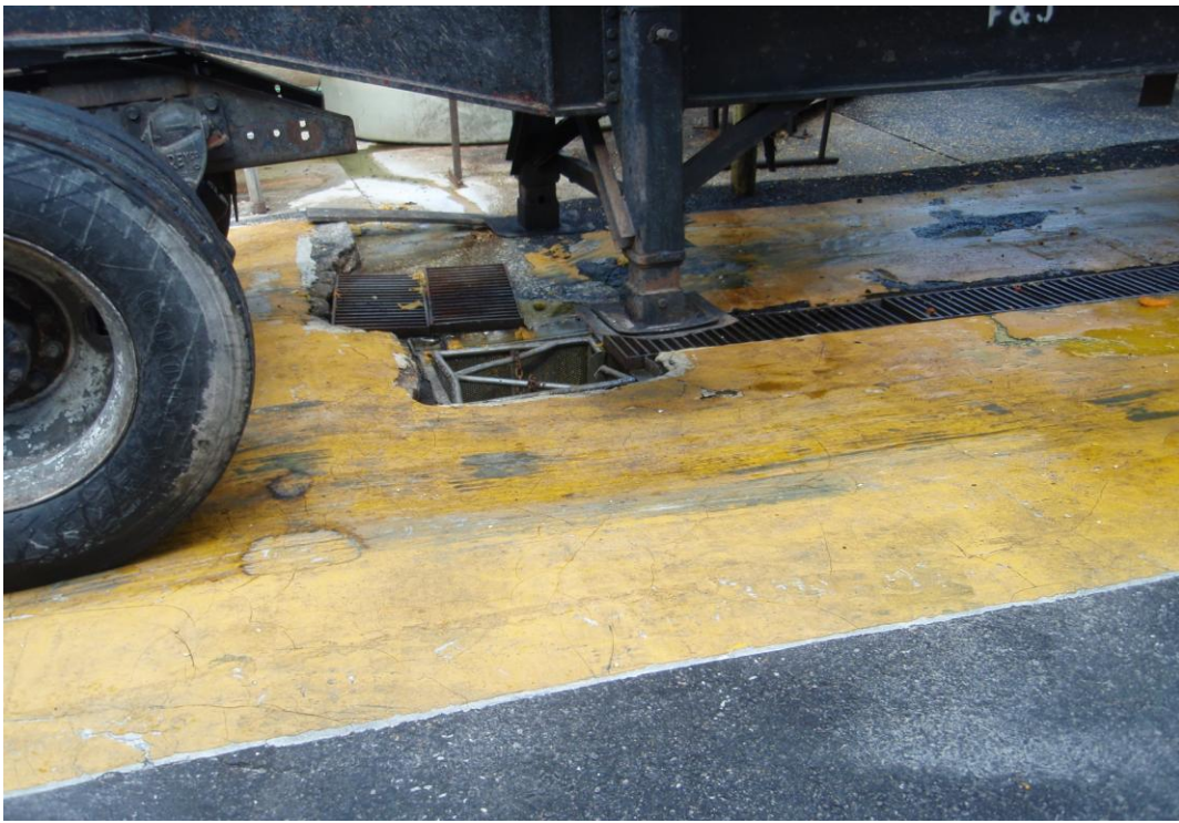
Drains catch the waste citrus products after being juiced.
