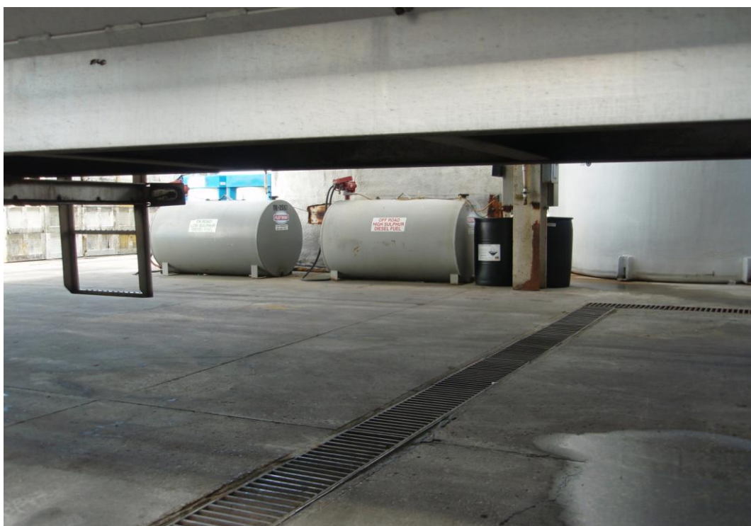
Two diesel tanks in the tanker area.
