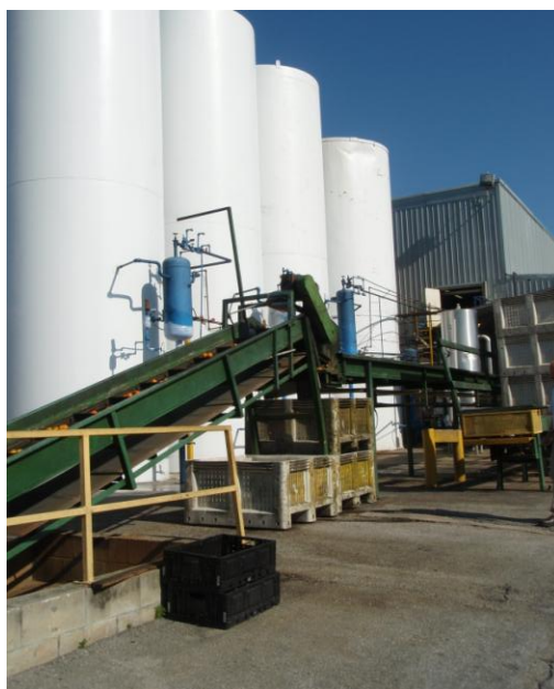
Ammonia tanks are located on the southern portion of the site, and are used by the juice plant for refrigeration purposes.
