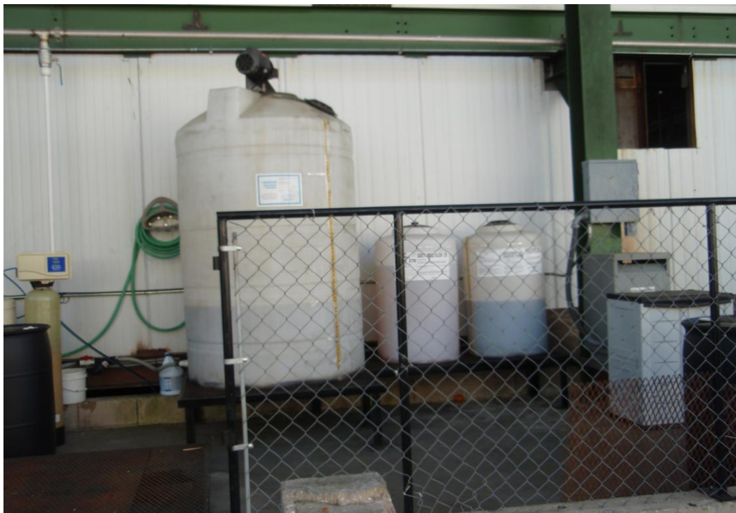
Fruit sanitizers, soaps, and waxes used in the fruit cleaning process are stored within a diked containment area on the western wall of the packing house.
